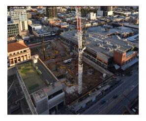
The project is in the process of transitioning from a civil excavation phase into a typical structure phase.
